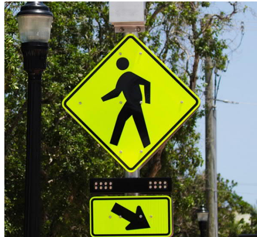
Figure 3.17: Rectangular Rapid Flashing Beacon
